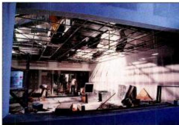
The CNN/SI facility under construction
